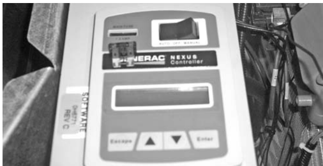
Figure 163. Remove 7.5 Amp Fuse
