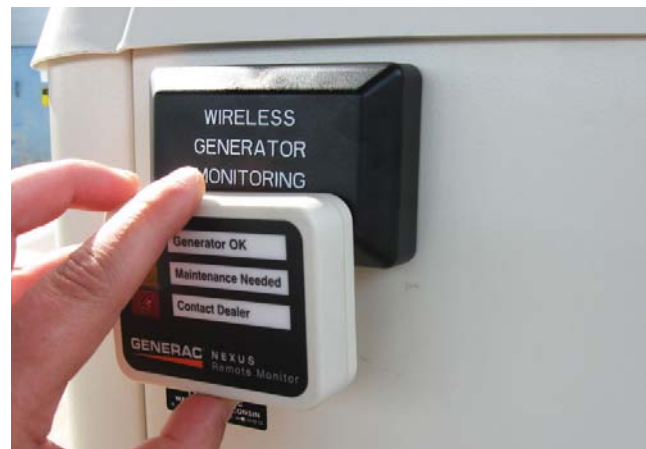
Figure 24. Place the Display Unit Against the Generator Transceiver
